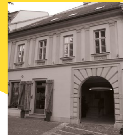
Burgher Town House at Trojičné námestie 5 in Trnava
